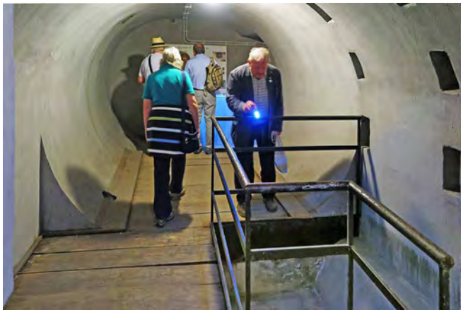
Mussolini's final bunker had a cylindrical cross-section for strength. This bay of the cruciform would have contained pumping machinery, never installed. Stewart Wild gazes into what would have been oil storage tanks if they'd ever been fitted
